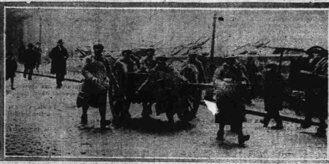
Upper—Under the watchful eyes of a French poilu, German workers loading coal destined to French consumption. Lower—Ammunition wagon being brought up to gun section.
