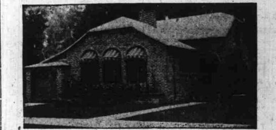
"The San Diego," hollow tile construction faced with rug or face brick.
