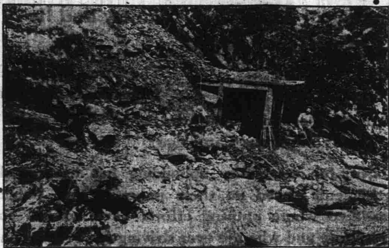
East Prospect Tunnel on Queen Vein, showing ore formation, width from hanging wall to foot wall about 130 feet. Showing exposed ore body.
