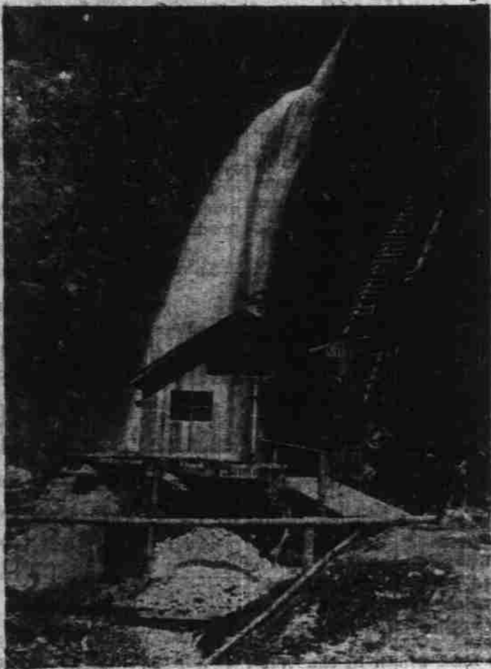
Power plant at Silver King Mines, at portal of main working and drainage tunnel.
