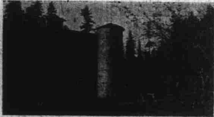
Silo Installation on Farm Owned by A. J. Schlecht of Tigard, Oregon.
