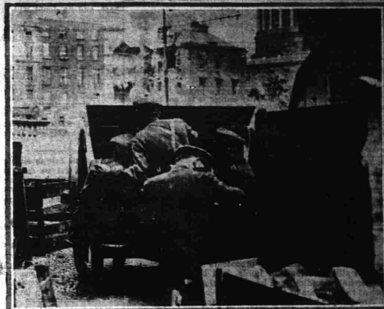
Free State artillery in action at Four Courts, where the rebel army was driven from stronghold by Free State troopers. The insurgents' losses were heavy, the tactics of the Free Staters, with their modern equipment and leaders, proving too big an asset.
