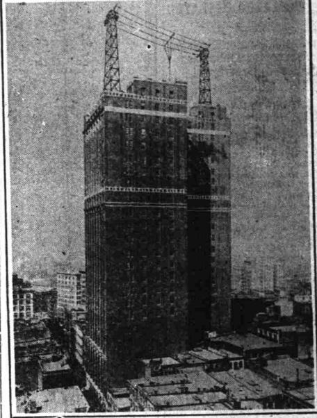
The largest commercial broadcasting station is near completion. It is the latest of the large and growing families of great radio stations devoted to the broadcasting of information and concerts. The plant is being constructed on the roof of one of the large buildings of the American Telephone & Telegraph Company and is capable of sending messages all over the country. The picture shows the station as it will look when the two towers of 100 feet are comleted and the "T" type aerial in place.
