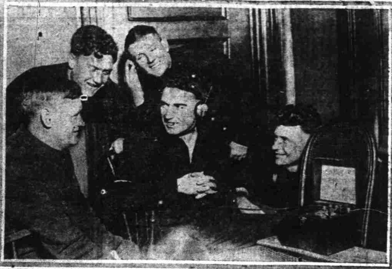
The radio telephone is the newest plaything. Both young and old alike find the small and compact apparatus amusing and at the same time instructive. Several cities throughout the country have installed the wireless telephone in their police and fire departments. Chicago set the precedent, and it did not take long for other cities to follow suit. Photograph, taken in Engine Company 15 of the Jersey City Fire Department, shows the smoke eaters getting an earful. They have a receiving set, and through this they hear anything that interests them. Some good joke is probably being wafted through the ozone and probably accounts for the smiles on their handsome countenances.
