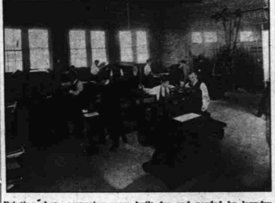
Printing shop—occupying room built for and needed by laundry.
