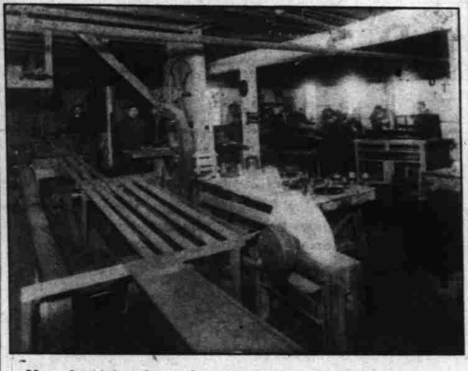
Manual training shop—shows congestion and inadequate light.
