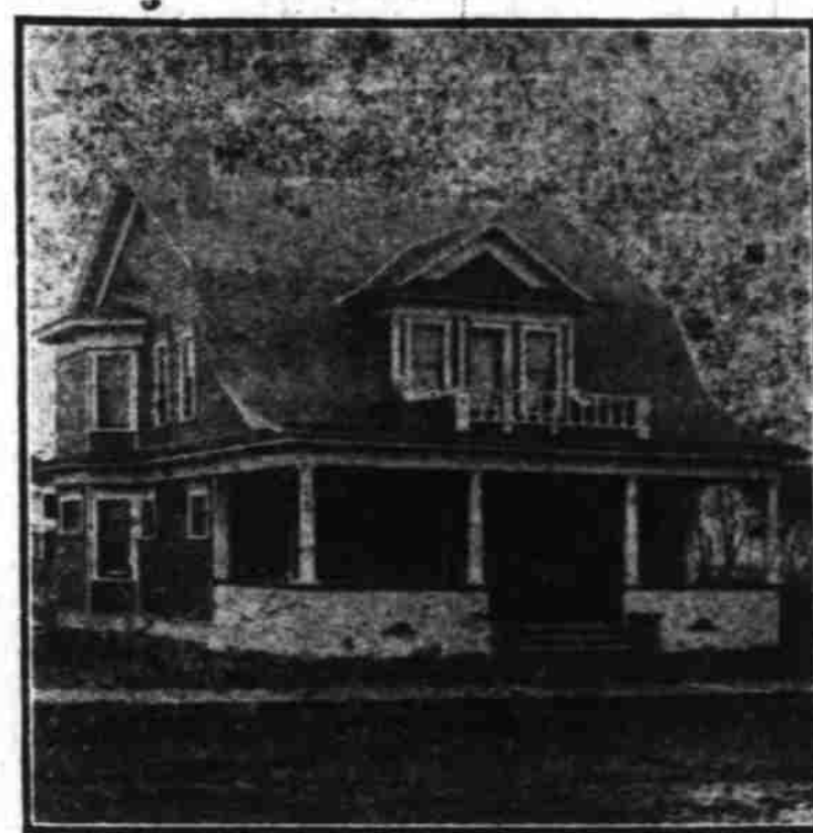
A Typical Stayton Residence.
