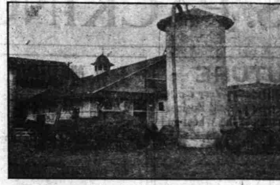
The Oregon Agricultural College Silo in Process of Being Filled.
