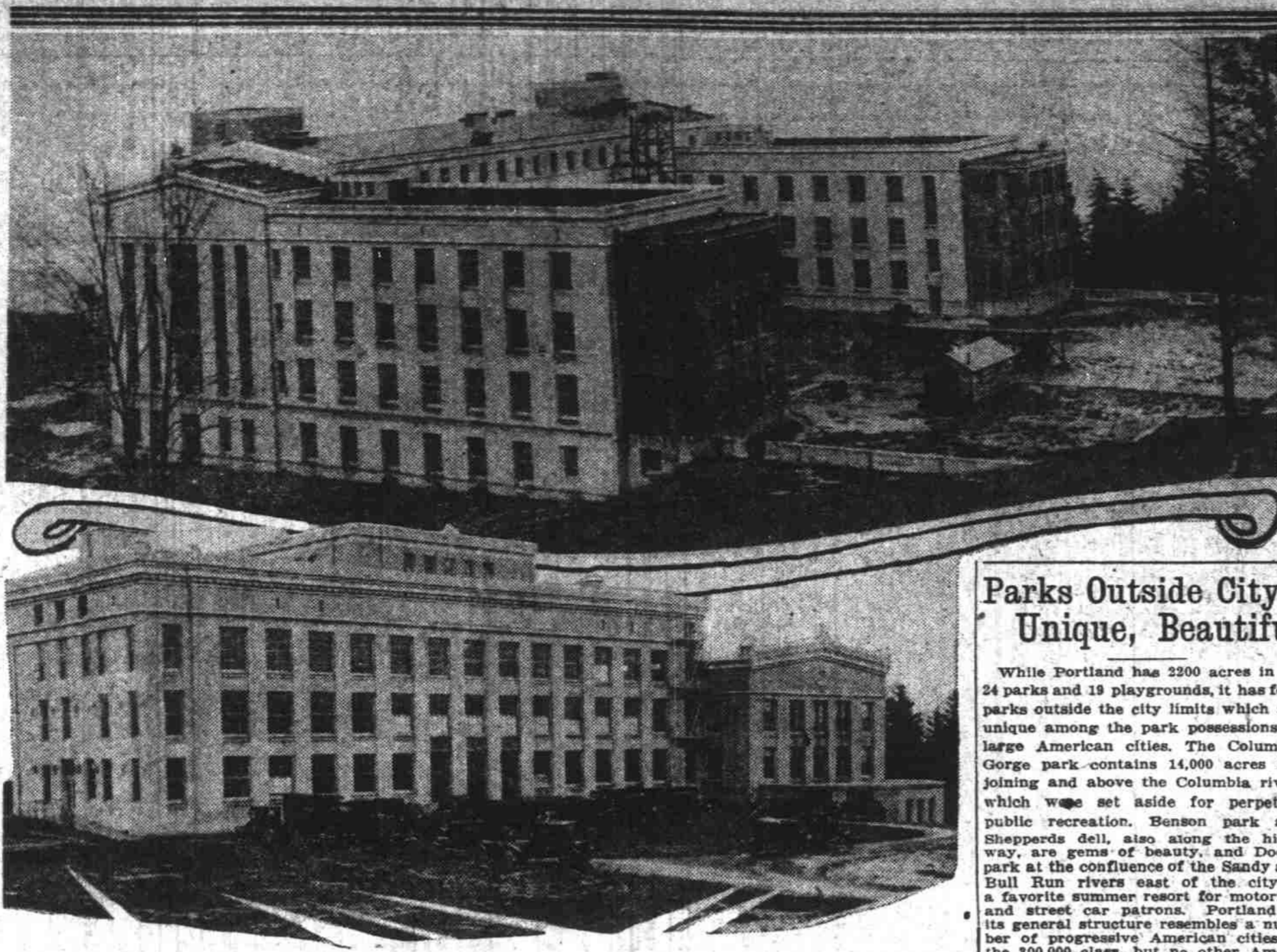
Above—New Multnomah county hospital nearing completion at a cost of more than $1,000,000, which will have 250 beds. Below—MacKenzie Hall, University of Oregon medical school, adjoining the county hospital, of which the middle wing was recently constructed.
