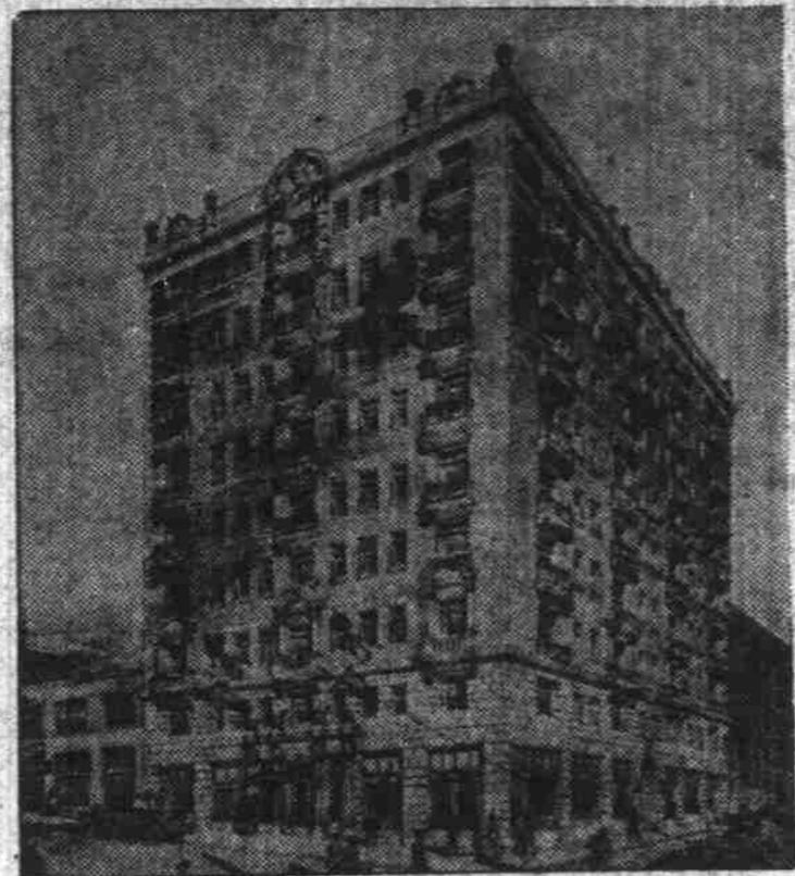
Everyone of its 72 apartments is equipped with a modern Electric Range
