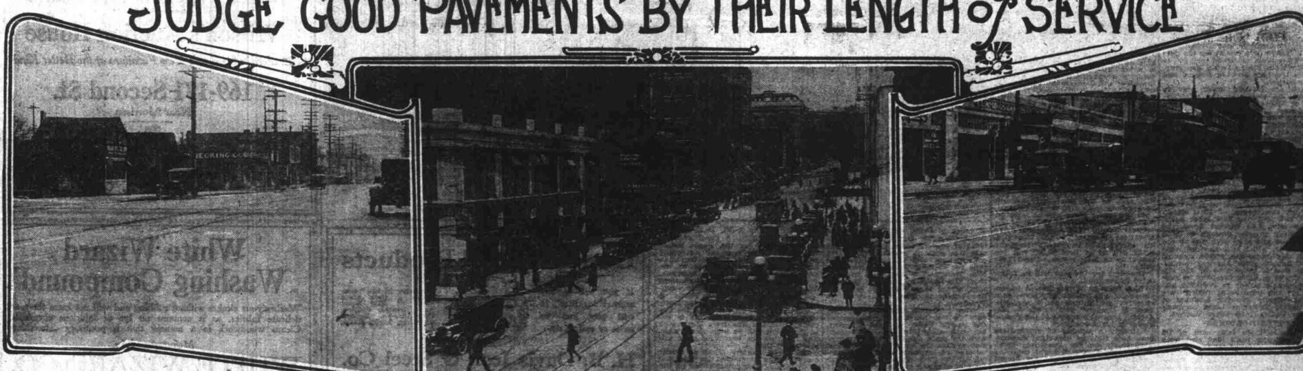
Grand Avenue Looking South from East Davis. Two-inch Warrenite-Bitulithic on Four-inch Compressed Crushed Stone Base. Constructed in 1907. Photo Taken November, 1922.
