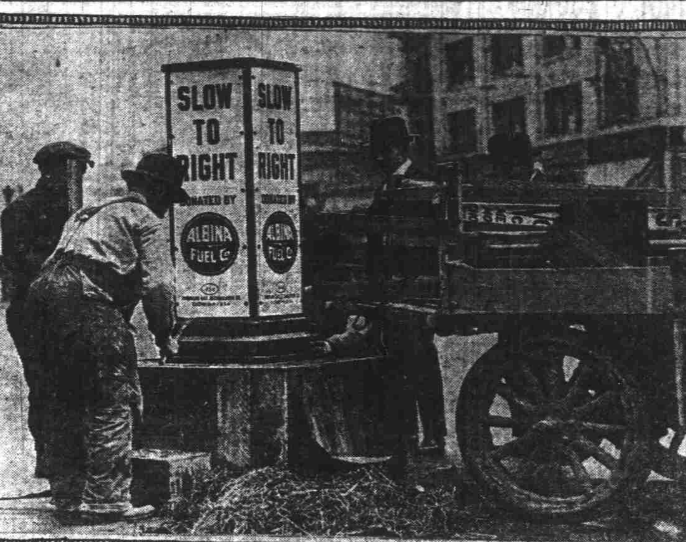
"Dry land lighthouses" erected at dangerous street intersections to warn automobile drivers. The lights are equipped with flashing acetylene burners. They were donated to the city by various business firms who have the privilege of using a space for advertising.
