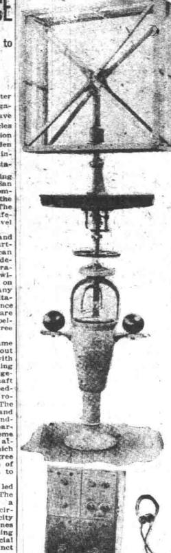
Above is the Kolster radio compass installed on a standard binnacle. Below is the receiver.
