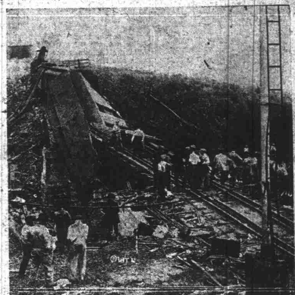
General view of wreckage at Sulphur Springs, Mo., which resulted from a collision on the Missouri Pacific between a fast passenger steel train travelling at high speed and a local made up of wooden coaches. The dead numbered 37, injured 127.
