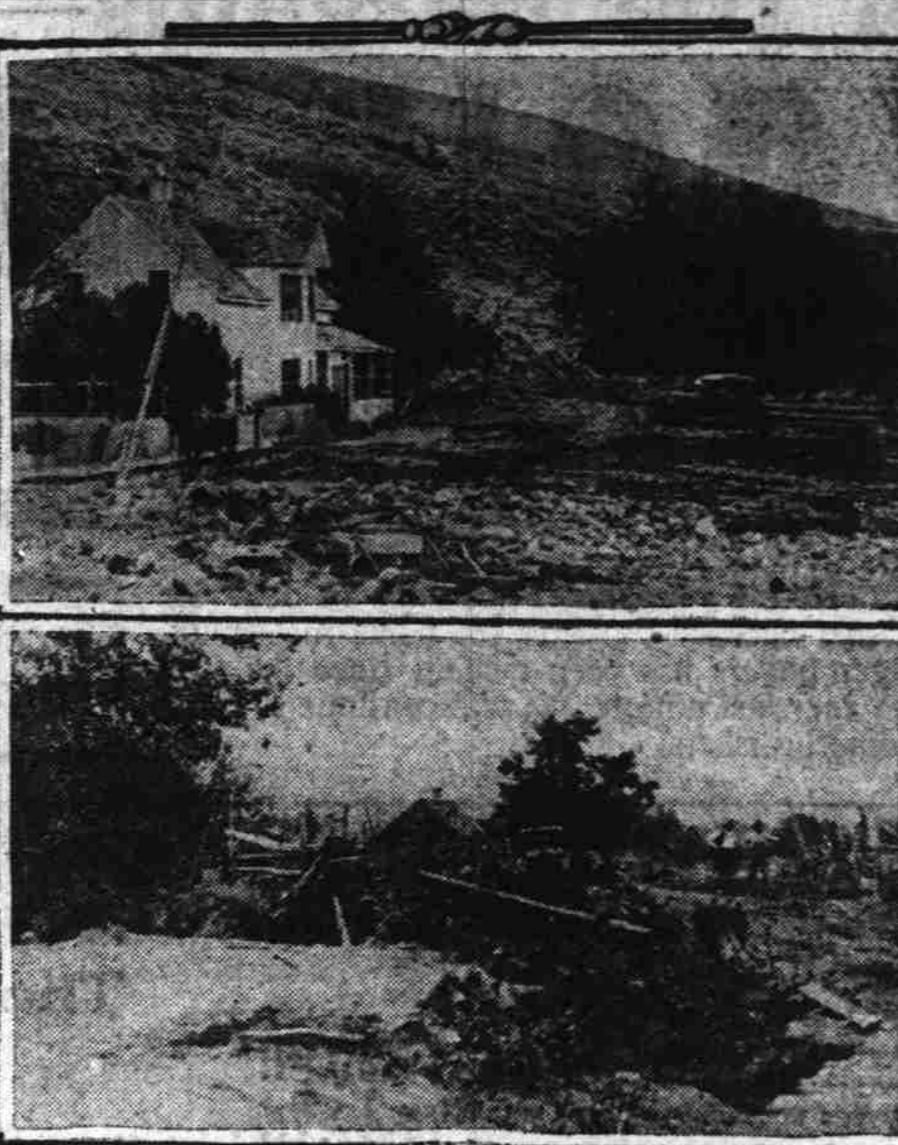
Above, residence of W. O. Cummings on the John Day highway; picture taken looking east along the highway. Rocks and mud filled the yard to a depth of two feet, almost high enough to get in through the windows. Only the quick work of the owner, digging trenches and building dikes of stone, prevented great damage to the house. Below, a washout on the highway west of Mount Vernon; temporary bridge shown in the lower right-hand corner.
