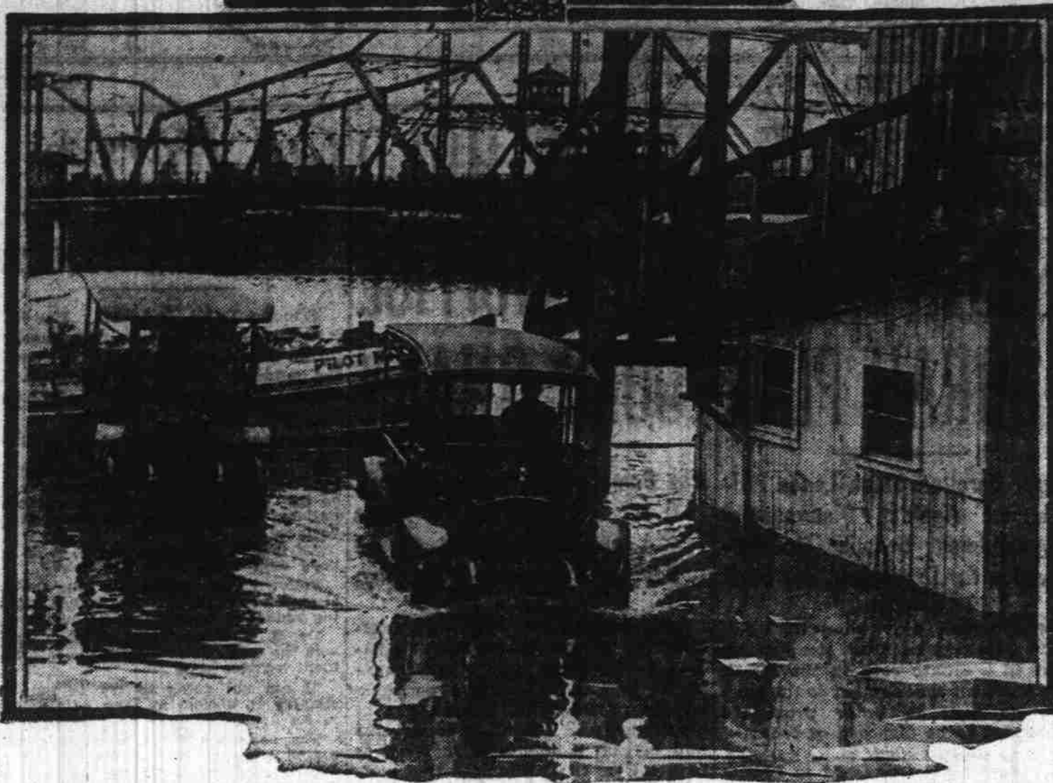
Scene at Alder street dock where truck drivers hurriedly unload milk cans from steamer and pull out just in time to prevent disaster to ignition system. Waters here have submerged lower dock levels and mount into runways where wagon traffic meets boat.
