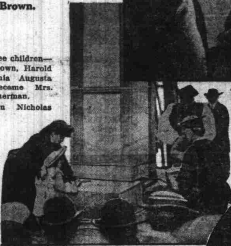
Baby Brown Laying the Cornerstone of the Brown Memorial Gates at Brown University, While the President and College Faculty Stand by in Their Official Robes.
