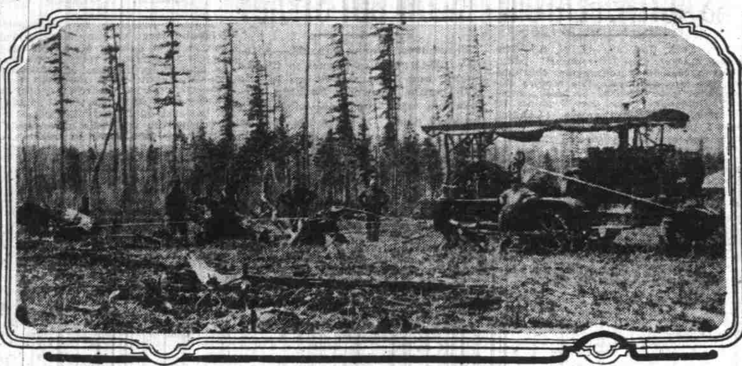
One of the modern machines that is making land clearing possible at less expense. The tractor is finding many uses.
