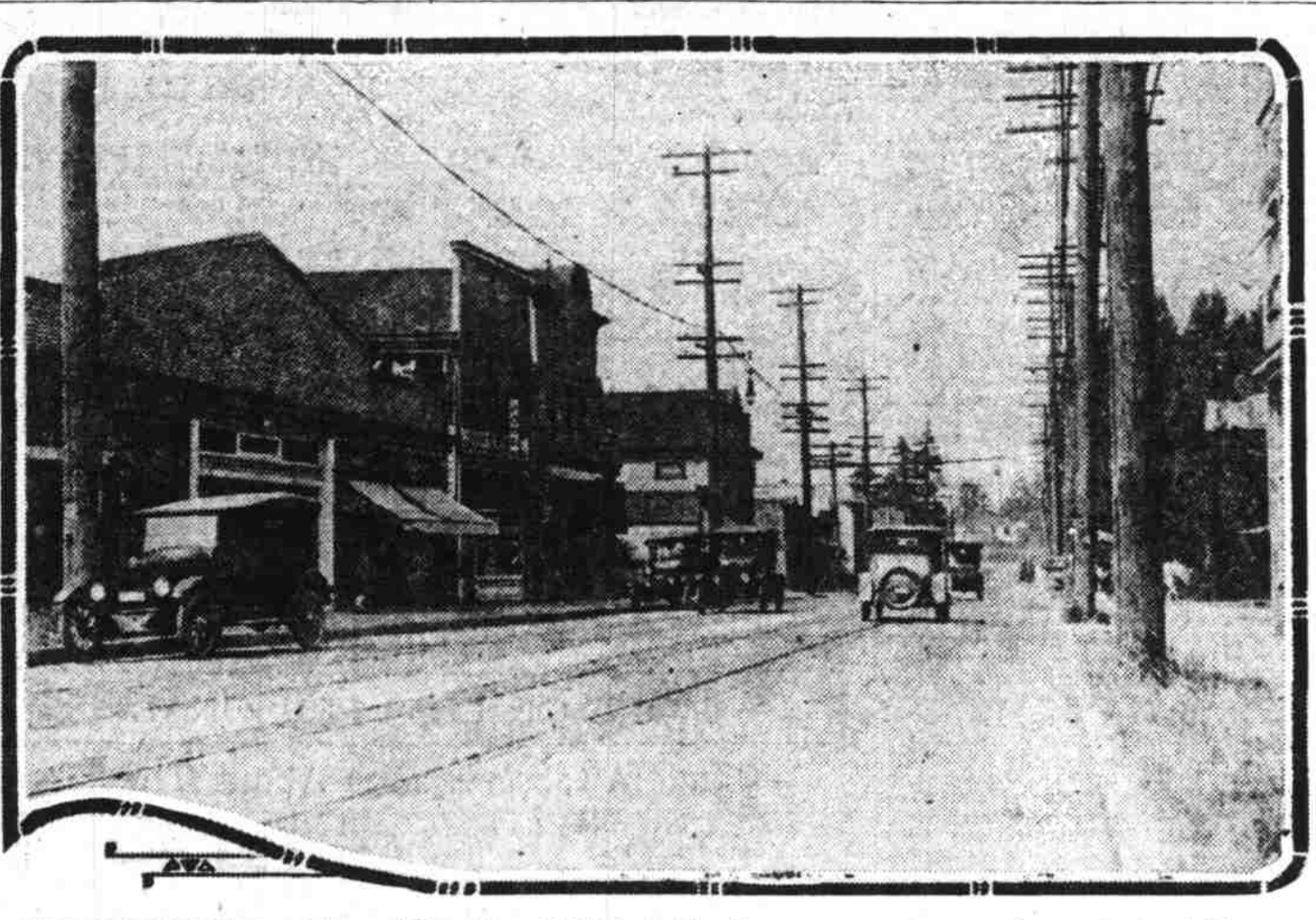
Along principal thoroughfare of Brooklyn district of city, shop center and scene of many industrial interests
