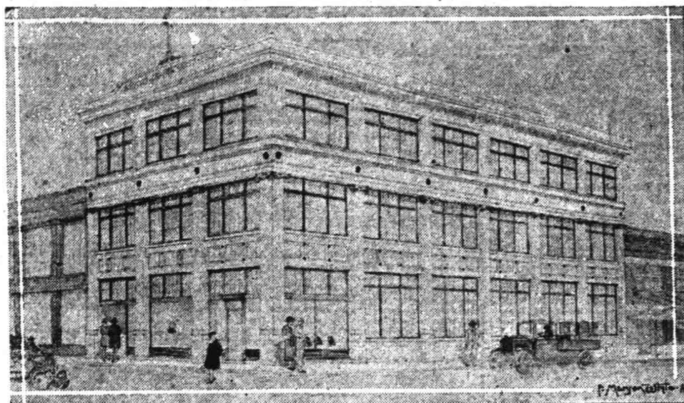
Reinforced concrete structure, 50 by 100 feet in dimensions, being erected for Morris and T. A. Binford at the northeast corner of Ninth and Couch streets. The entire building will be used for printing and allied graphic arts.
