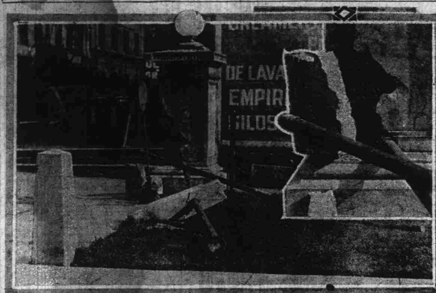
Wreckage of concrete rail around municipal landing at Stark street, where driver crashed through with idea it was Morrison street span.
