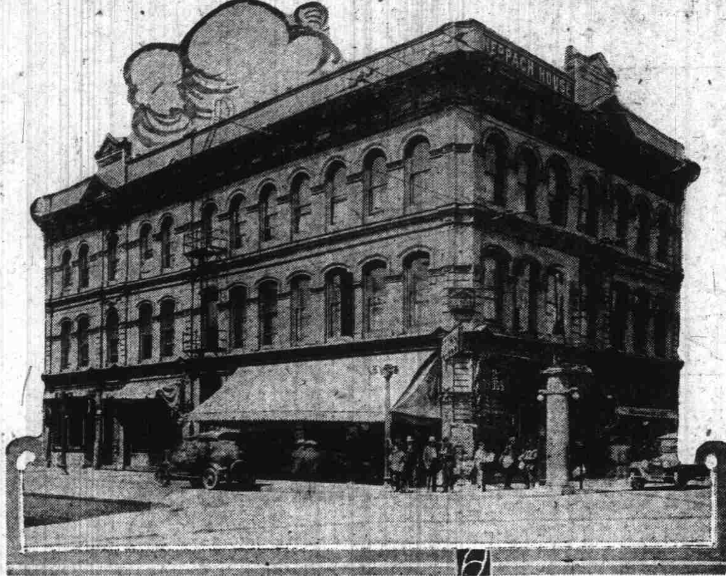
Three story structure at the northwest corner of Third and Burnside purchased last week by Dr. Sol Miller. The building was erected 35 years ago and was considered one of the finest structures in the business district at that time.
