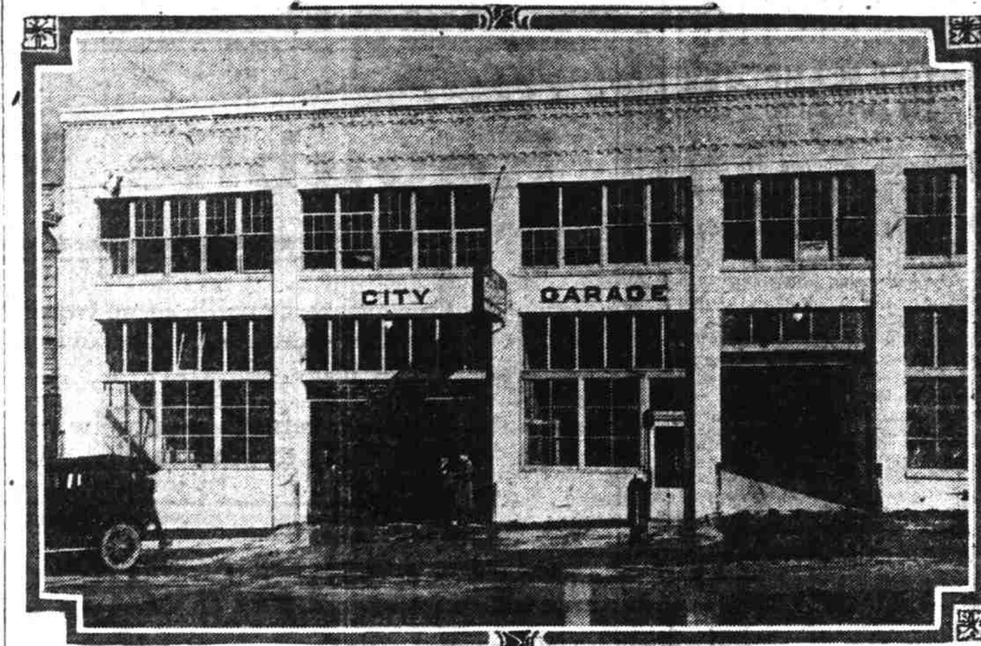
The new building recently occupied by the City Garage is one of the most modern and complete now in the service of the city's motoring thousands. This building, at Twelfth and Alder, was erected at a cost of $35,000 by the Portland Elks and occupies one of the most valuable lots in the city.
