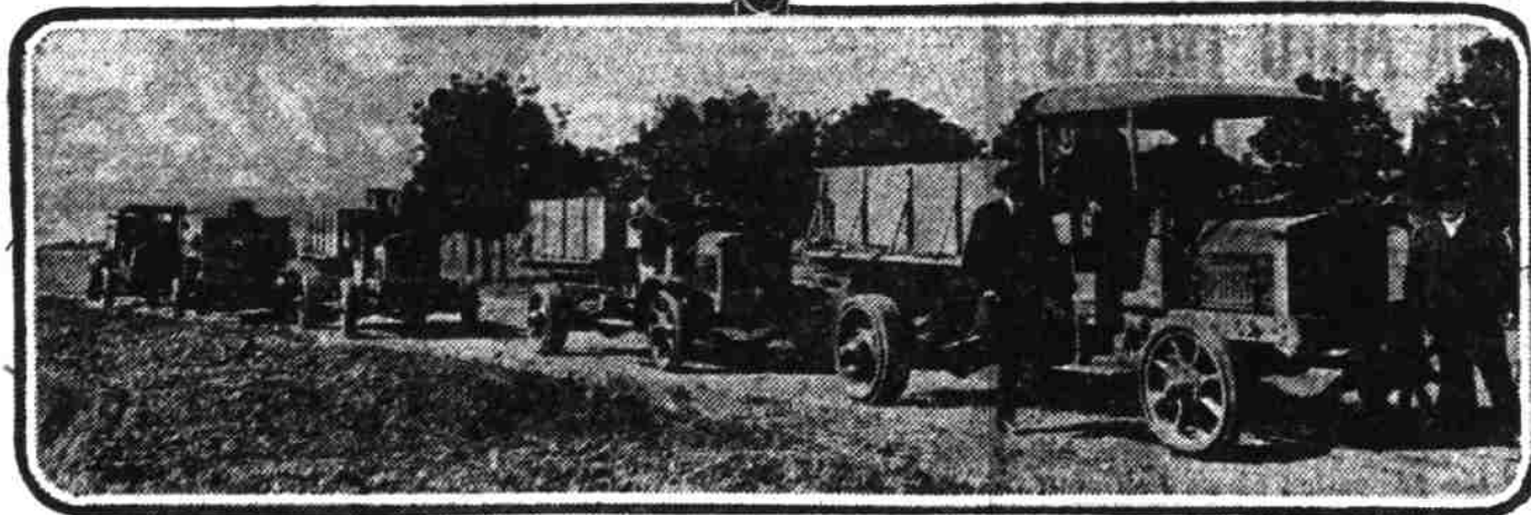
Fleet of Federal trucks equipped with Firestone tires, used for road work and dump-hauling near Medford. Or. Del Wright, manager of the local branch of the William L. Hughson company, Federal distributors, is standing at the extreme right.
