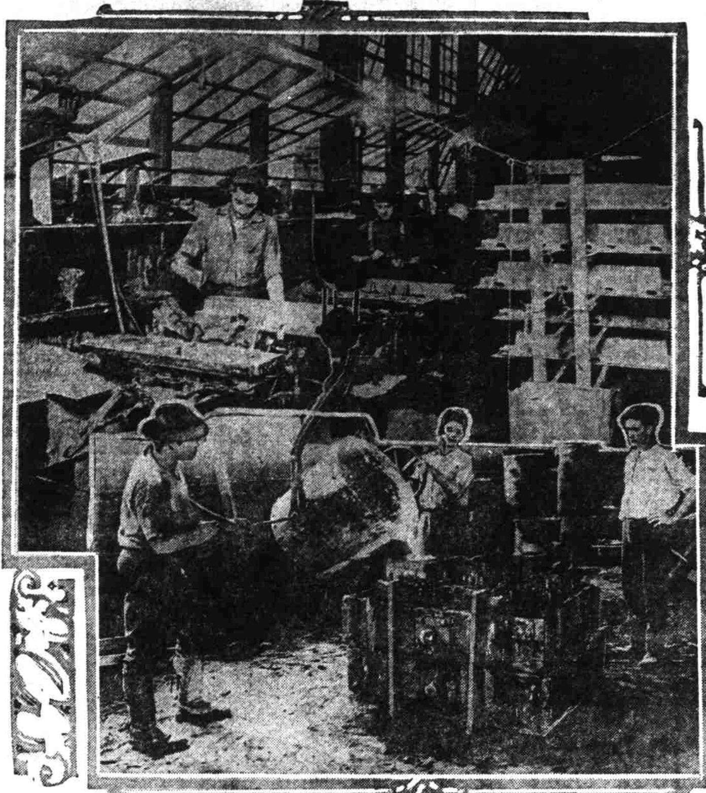
A hot spot in the foundry where the cylinder blocks for the Chalmers Hot Spot Six are turned out. The top view shows the careful work and the skill required in forming the sand moulds of the cylinder block. The lower shows the molten metal being poured into one of the huge cores on the foundry floor.
