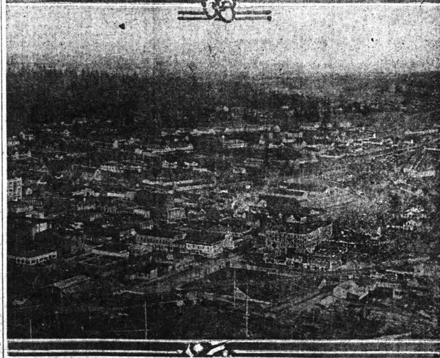
General view of U. S. military reservation at Vancouver with section of city's business district in foreground
