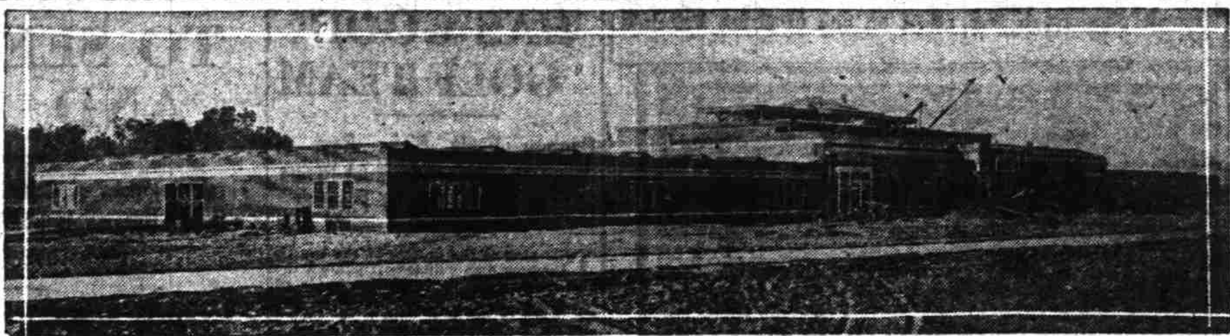
Latest photograph of new exposition buildings, taken Friday. Over 200 men are now rushing the work to completion.
