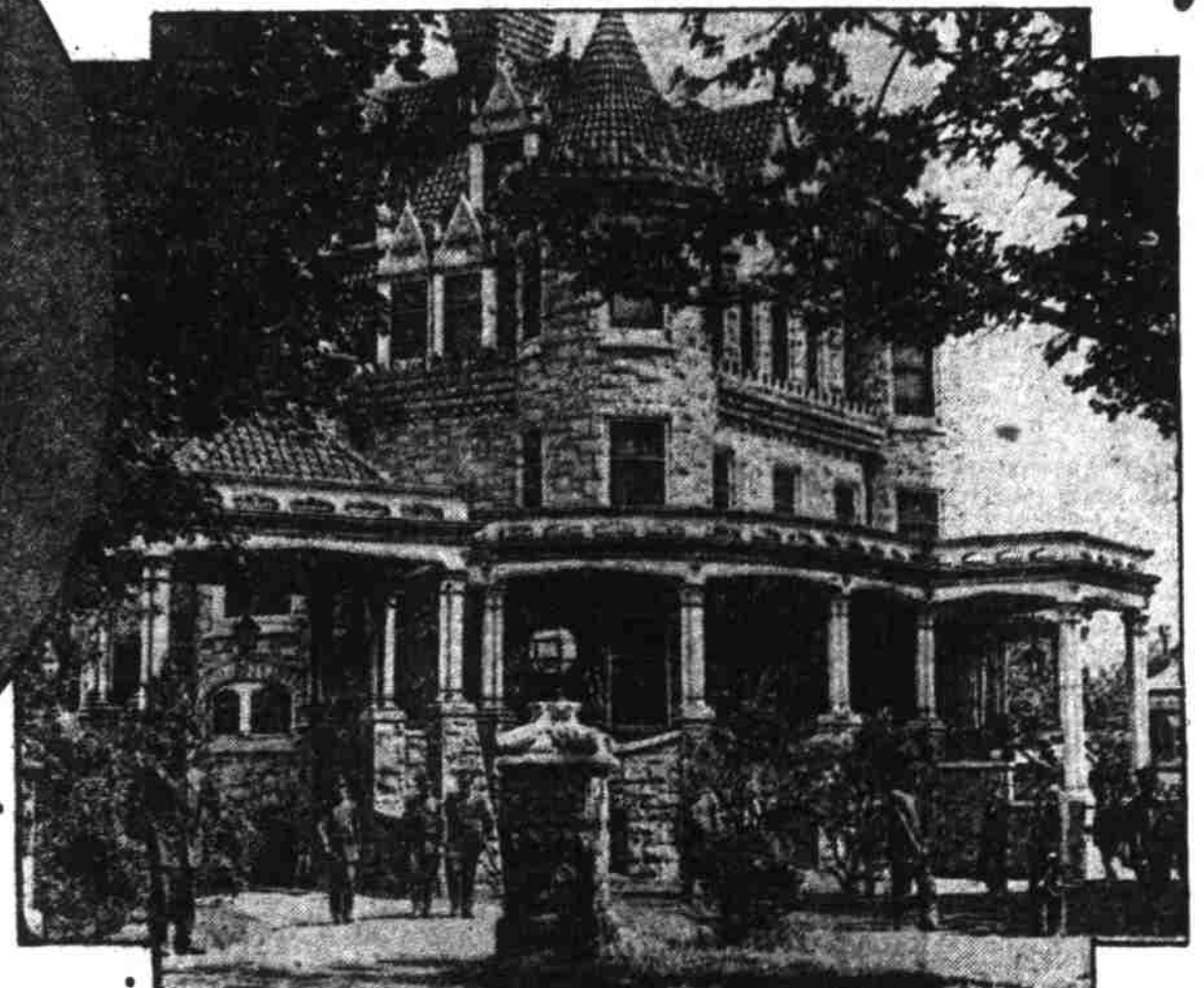
The Bergdoll Home, Near Philadelphia, Surrounded by the Cordon of Police on Constant Watch for the Return of the Brothers.
