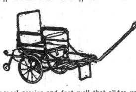
Full collapsible sulkies with 14-inch reclining back. Leatherpadded spring 10-inch wheels 3/8-inch rubber Combination
