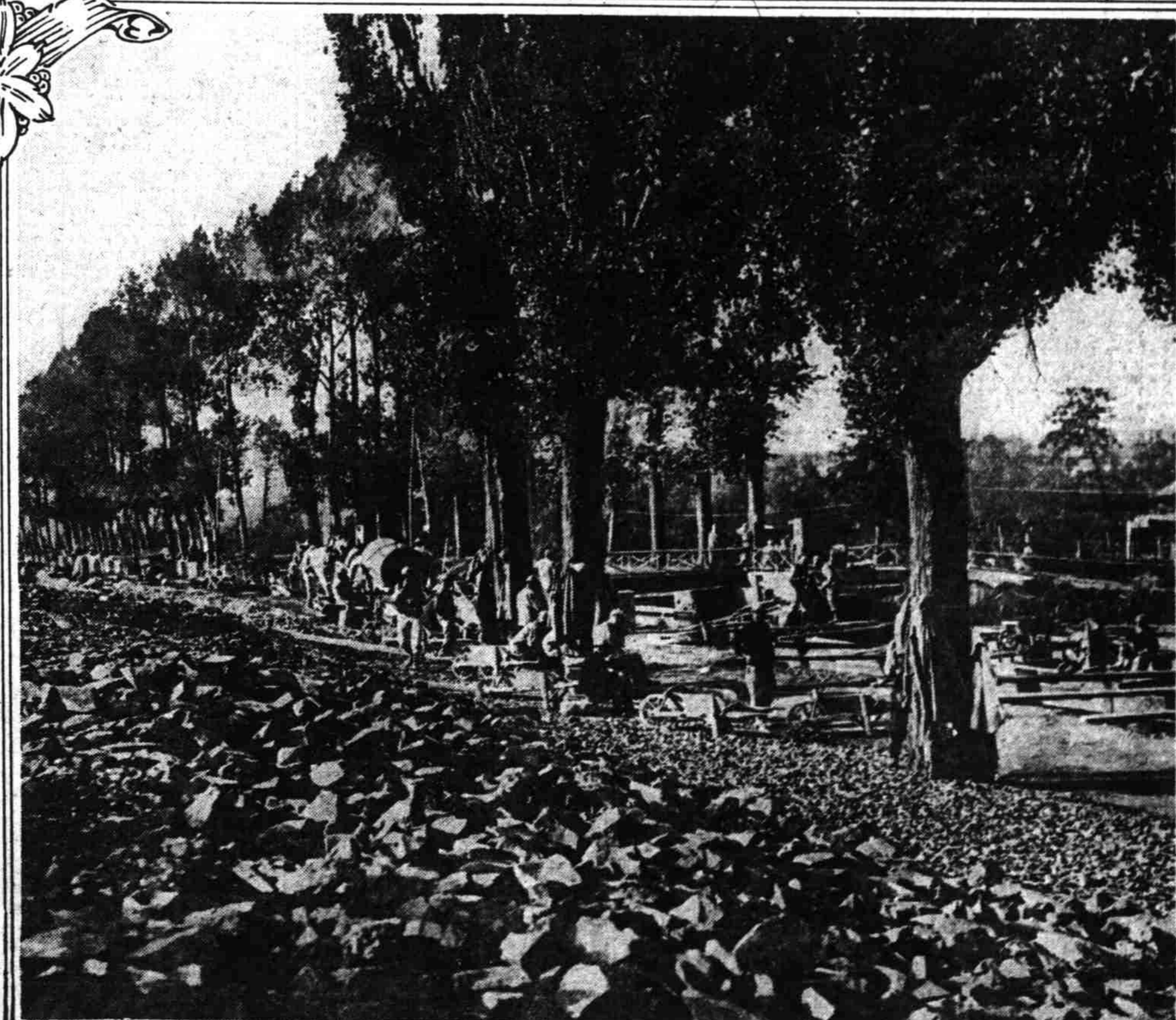
French soldiers building military roads behind the lines in the Somme. The stones for the roads are brought up by canal barges, and though the cost is great in labor and material, it is as nothing compared with the vast military value of good highways in times of battle, when all depends upon moving great numbers of troops to fill the gaps with the least possible delay.
