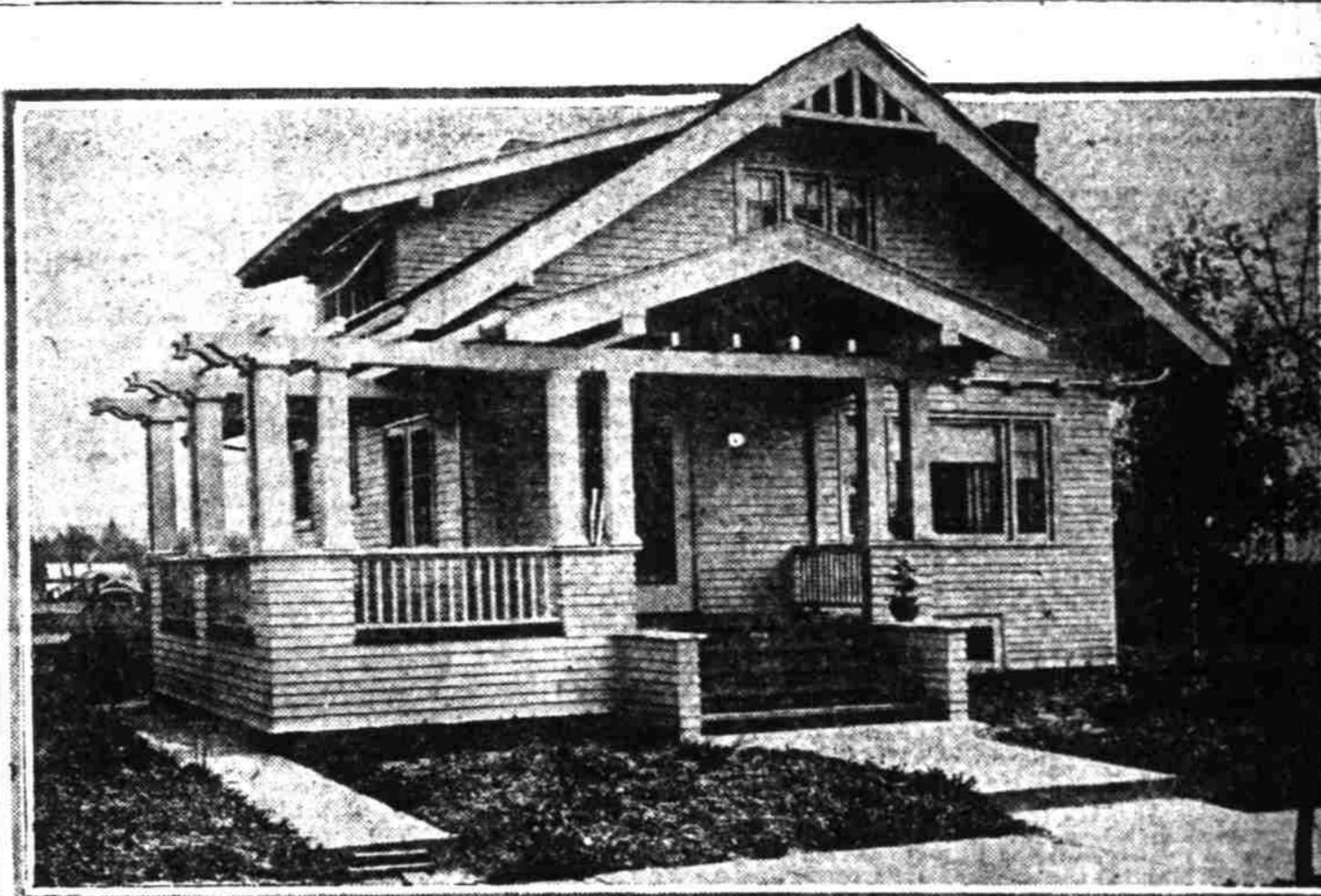
Above—Home of Mrs. A. B. Spinney, 1256 East Nineteenth street. Below—Brown residence at East Eighteenth and Bybee streets.
