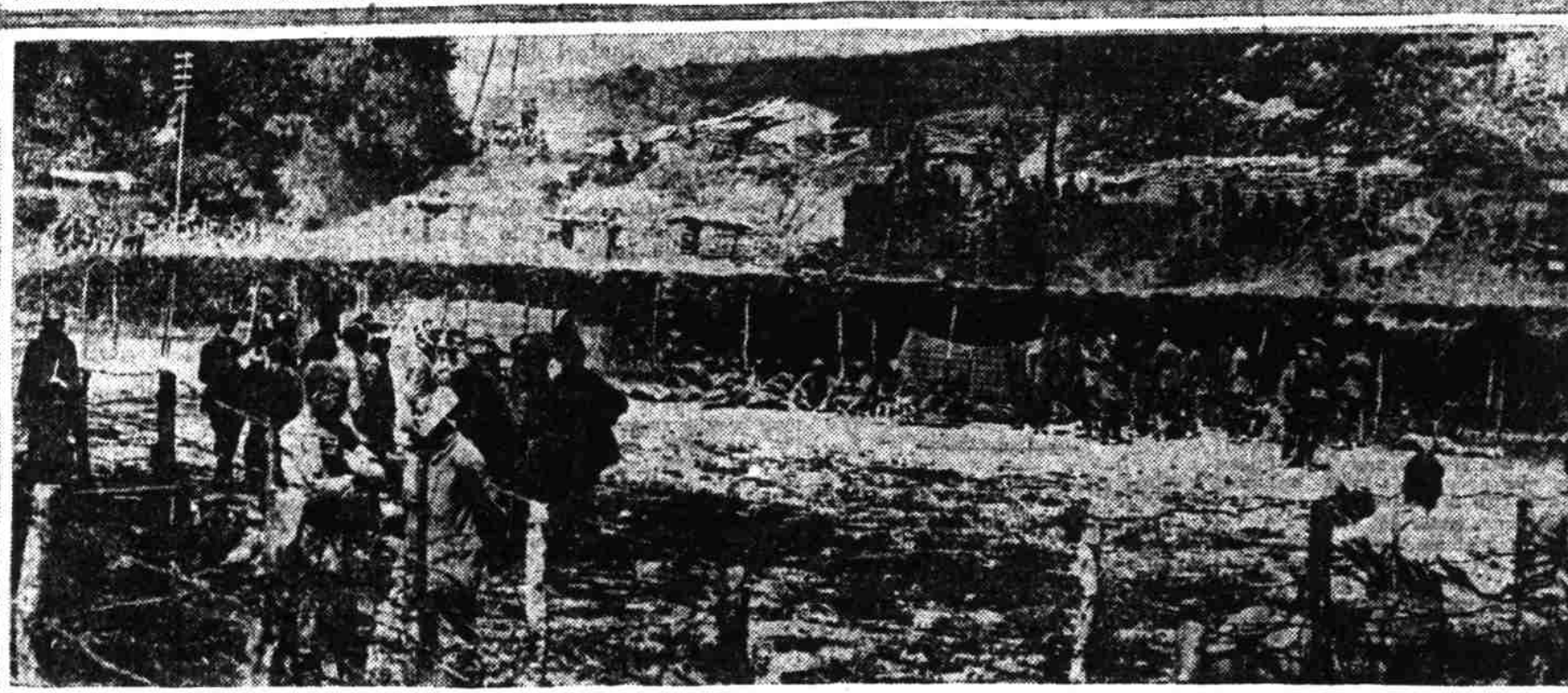
Top—Prisoners resting while being marched back behind the lines. Germans in prison camp in foreground. Background is what is evidently portion of English second line trenches. British soldiers have built dugouts in hill and protected them with sand bags. These pictures are issued by the British official press bureau.
