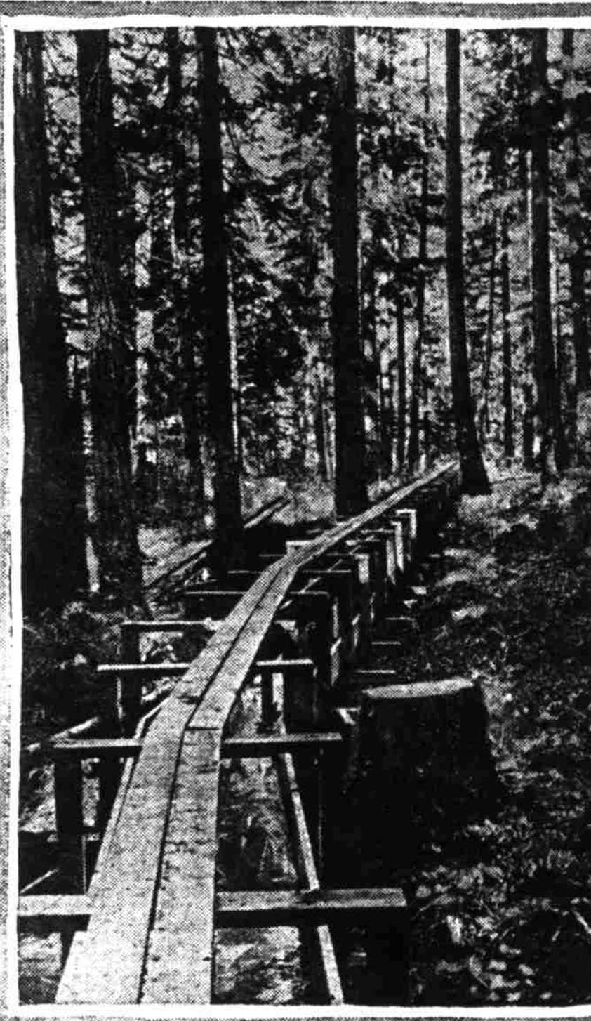
Part of the flume at the new Butte falls fish hatchery.
