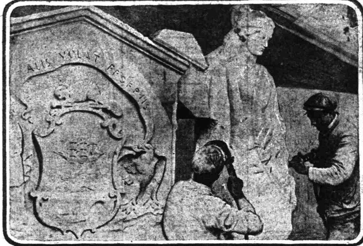
Detail of Process of Carving Life Sized Figures and Copy of State Seal Above Main entrance to new home of First National at Fifth and Stark Streets.
