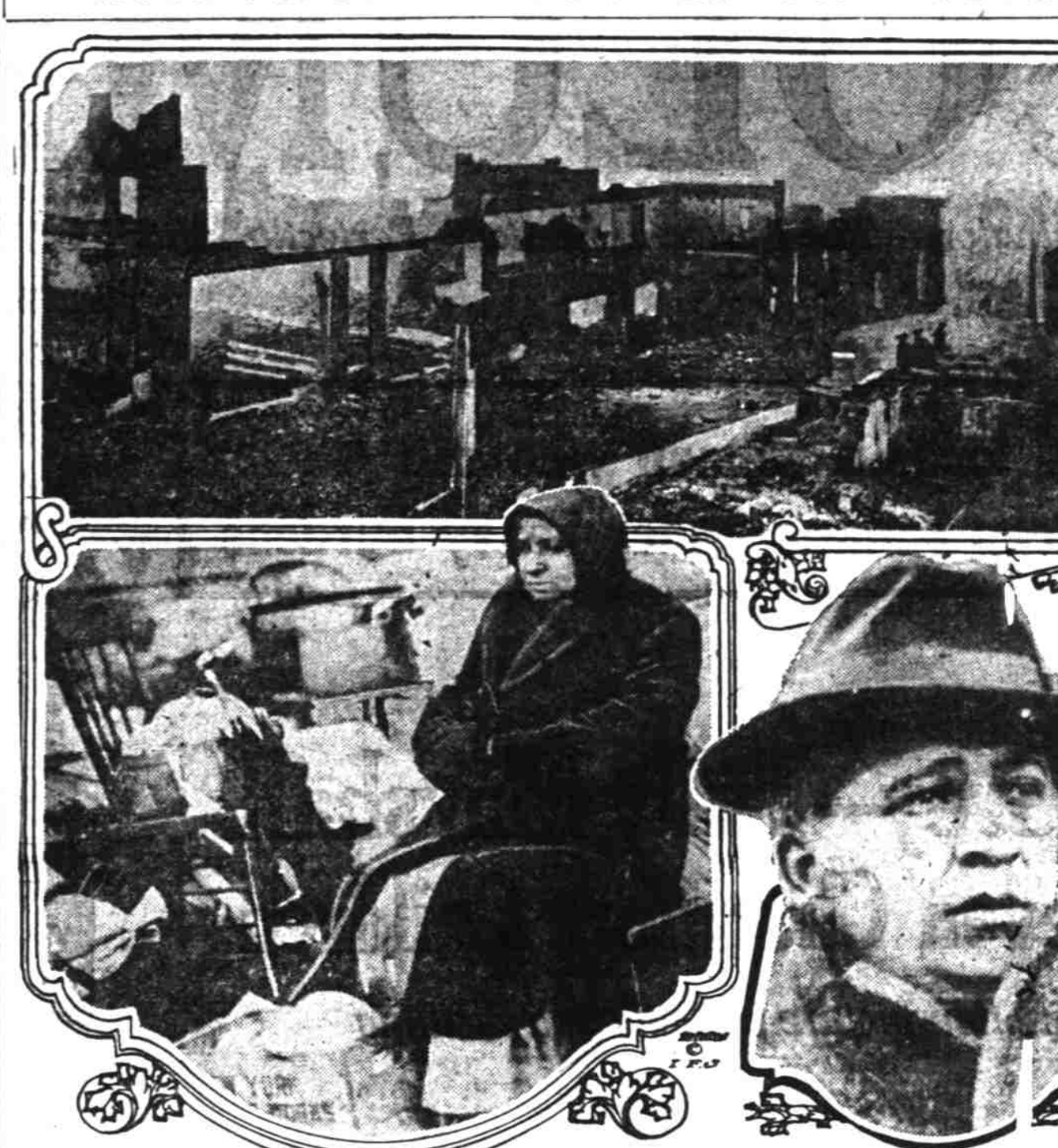
Above—Ruined section of East Youngstown, Ohio, where rioters levelled the business section and looted the wreckage. Below, left to right—Mrs. Stephen Kovic seated among the household goods saved from her home wrecked by rioting strikers; Mayor W. H. Cunningham among the ruins.
