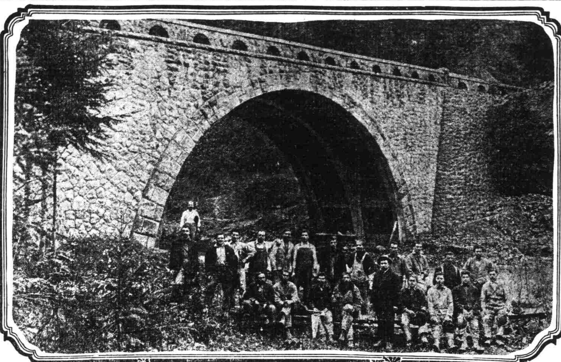
The Eagle creek bridge on the Columbia river highway near the Hood River county line, which has just been completed. It is a combination of the ancient stone arch and modern concrete construction. The weight of traffic is supported by the concrete and the stone veneer gives it its beauty. The span is a 60-foot arch and the length of the bridge over all, including abutments, is 140 feet. The bridge deck is 40 feet above the stream. The cost of construction was approximately $10,000.
