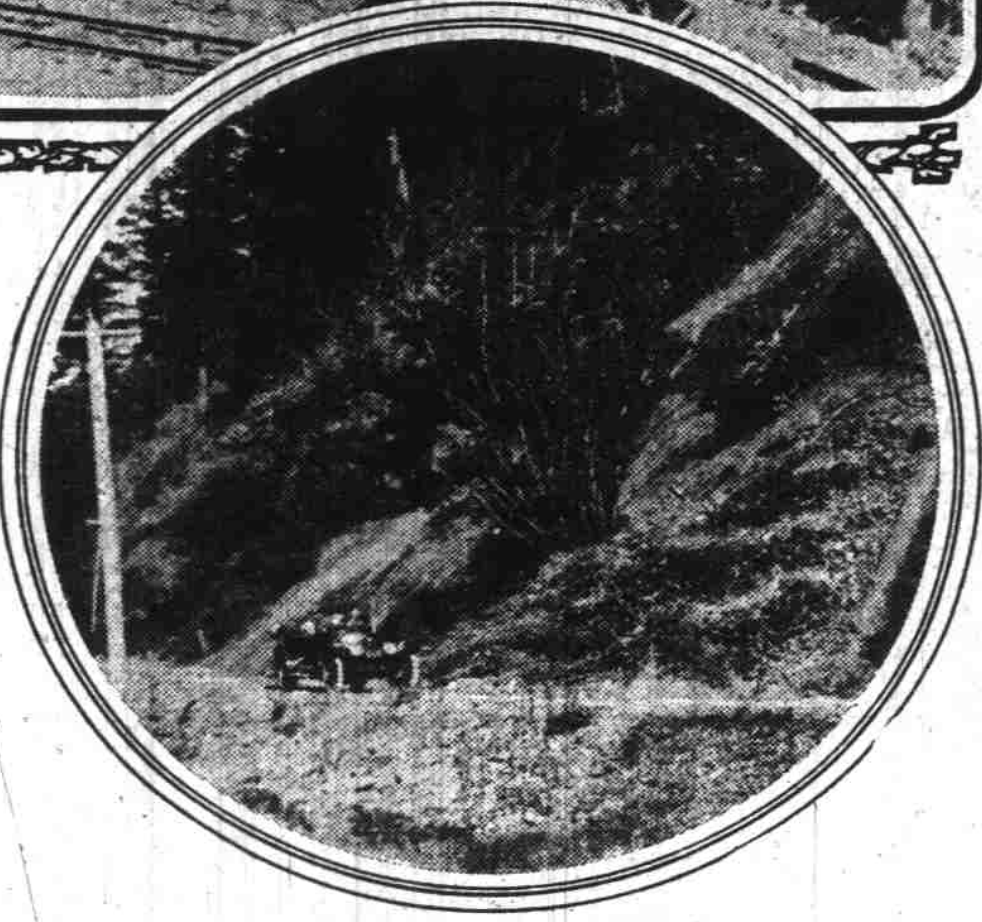
Top—New road and new bridge across Sandy, near automobile club. Bottom—Earth slide.
