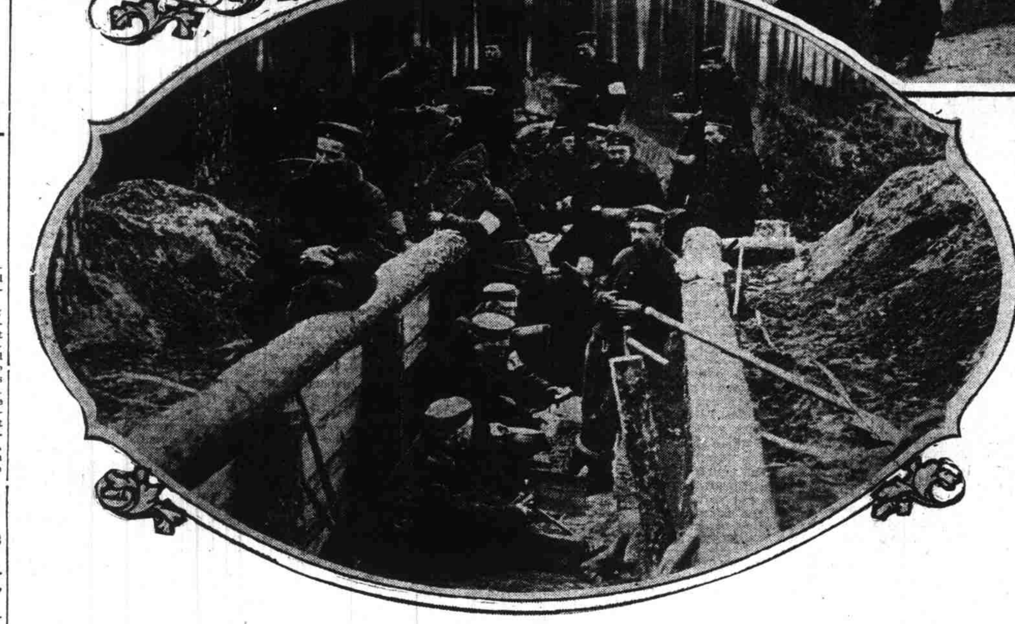
Top, left to right—Two German soldiers in East Prussian region occupy an old wagon abandoned by the Russians. A factory building in the suburbs of Paris wrecked by a bomb dropped from a Zeppelin. Bottom—German soldiers in Poland engaged in trench building operations, pause for their noonday meal.
