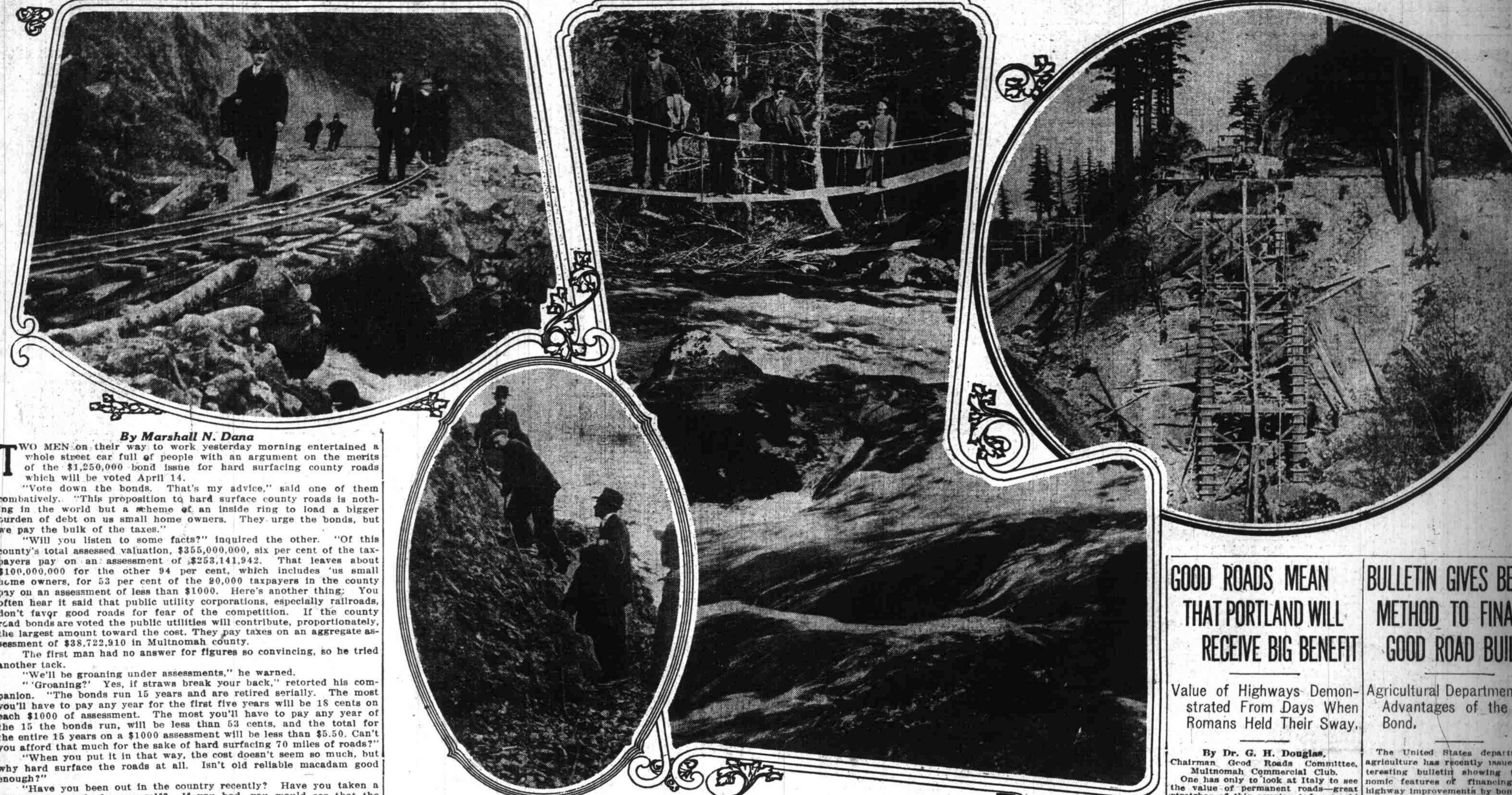
Top, Left to Right—How the construction goes along face of cliff near Multnomah county-Hood River line. The swinging bridge over Eagle creek, which is to be replaced by a 24-foot-wide span of native, hewn stone; swirling water of Eagle Creek beneath the bridge. Bottom—Climbing by rope ladder over the basaltic columns that must be cut away to permit the Columbia River Highway to circle the south pier of the Bridge of the Gods.
