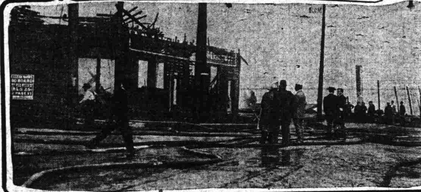
Top—Coonrod rooming house, which was damaged. Bottom—King-Fisher Mattress Works building, which was destroyed.
