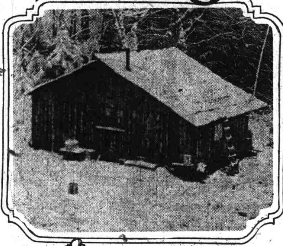
Top—Picture taken just after completion, before the brush was cleared away. Bottom—In the winter time, showing the clearing about the cabin.
