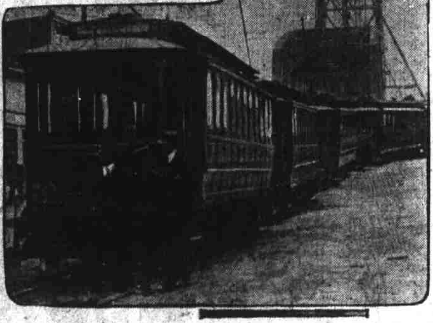
Picture shows draw while out of Commission and delayed cars at west end of span.
