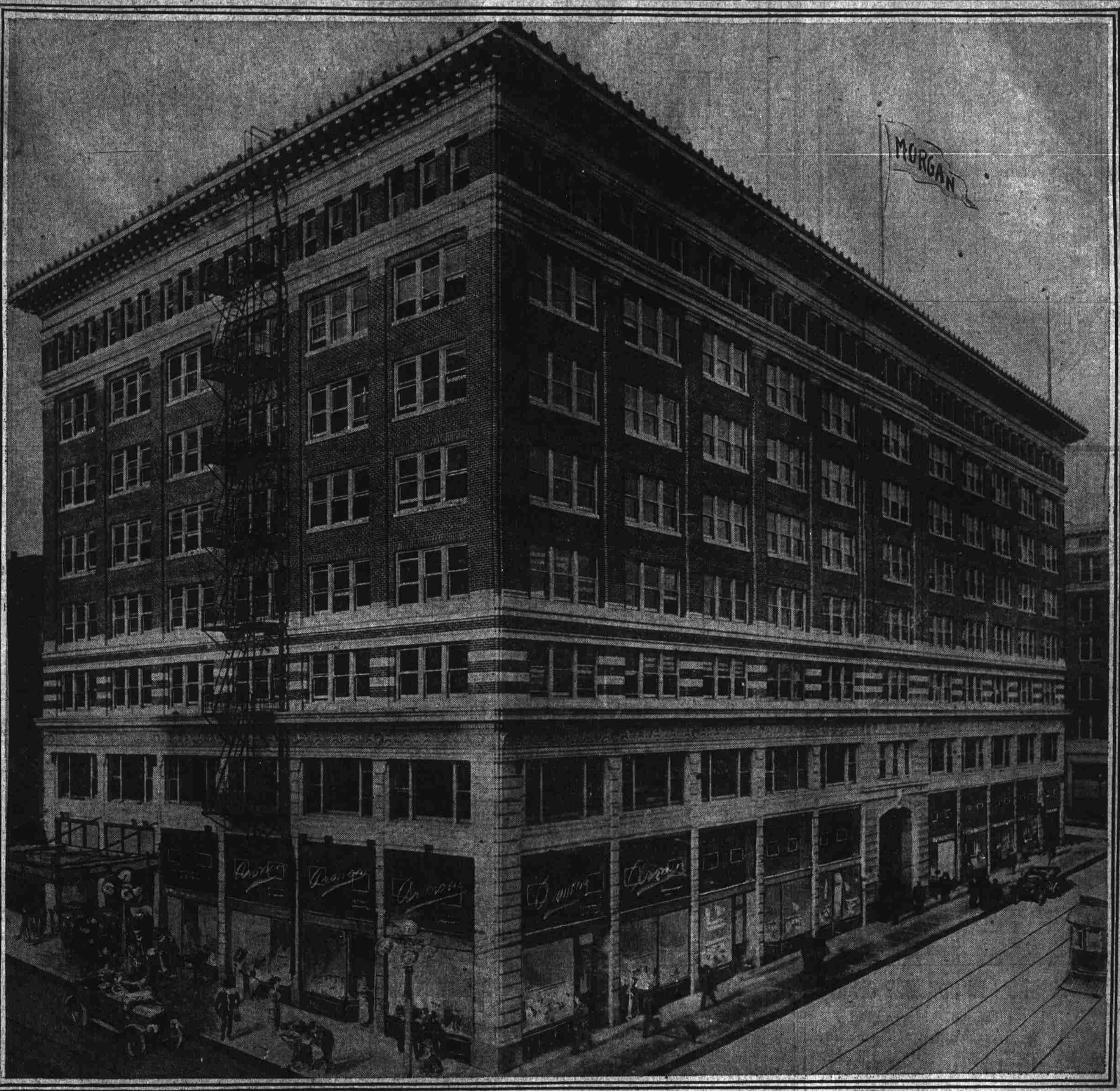
This new office structure, which graces upper Washington street, occupies an entire half block on the south side of Washington street, between Broadway and Park. A time record was made in its construction. Work of demolishing the frame structures which formerly occupied the site was begun January 21. Today, after an interval of a little more than eight months, the building is occupied.
