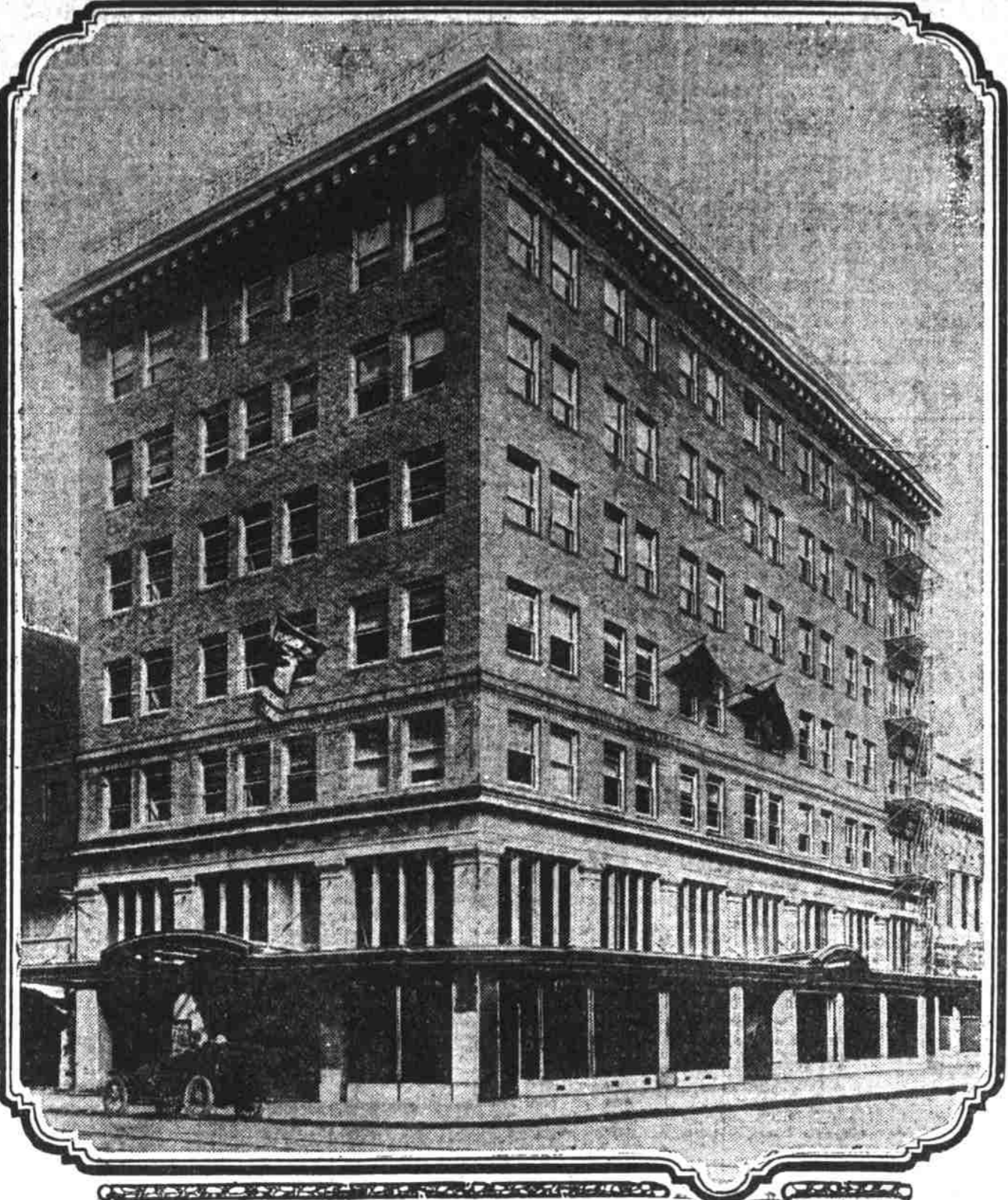
Newly completed Panama building.
