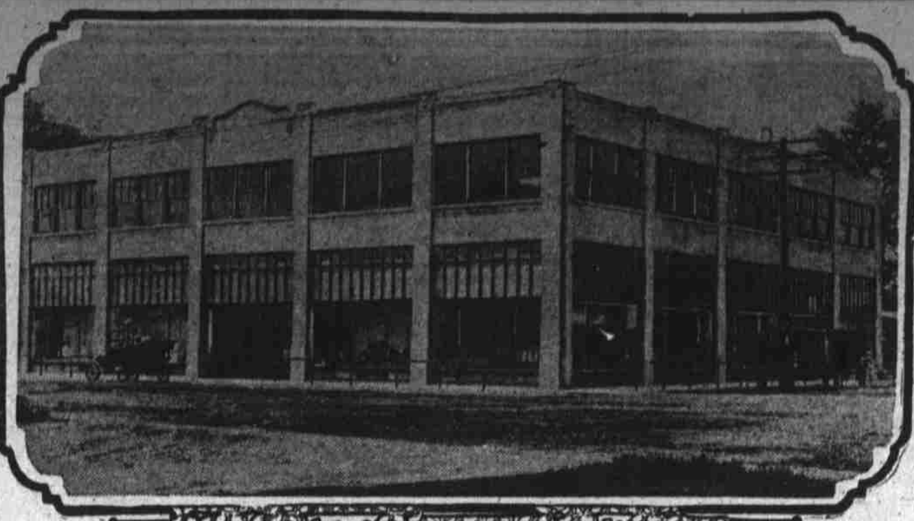
New Carleton & Rosenkrans store, which is of reinforced concrete.
