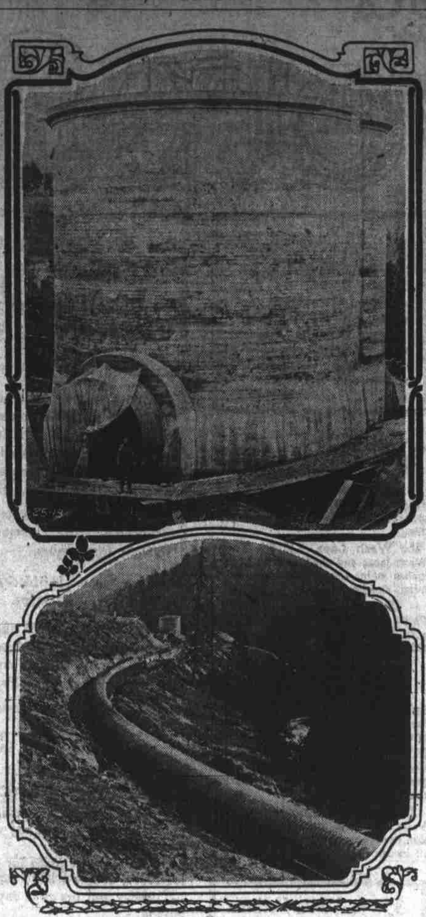
Views of huge water conveyor at Northwestern Electric company's plant on White Salmon river. Top—Forebay, or surge tank by which flow of water is controlled. Bottom—Section of pipe leading from dam to power house.
