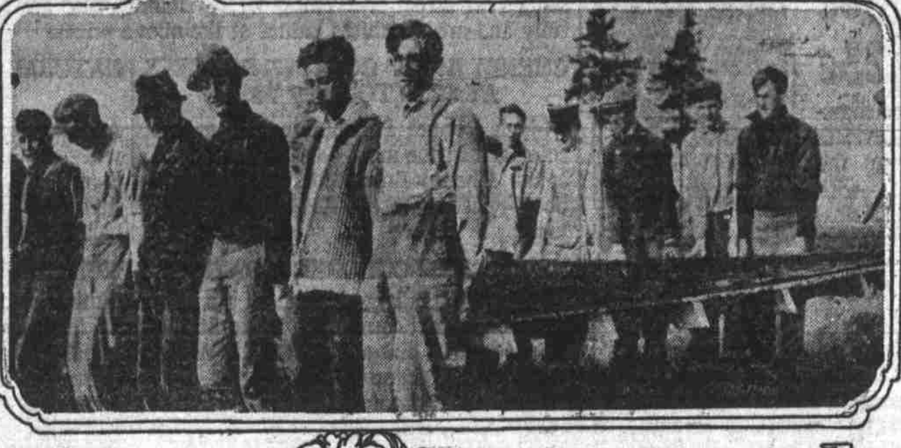
Top—Reed College girls on Campus Day. Center—Men removing shed to new site where it will serve as a boathouse. Bottom—Boathouse roof on the move.
