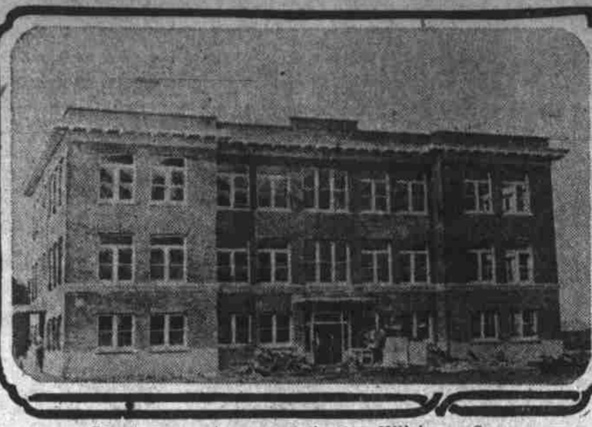
Structure nearing completion at Hillsboro, Or.
